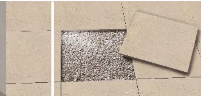
DRY INSTALLATION GRAVEL
